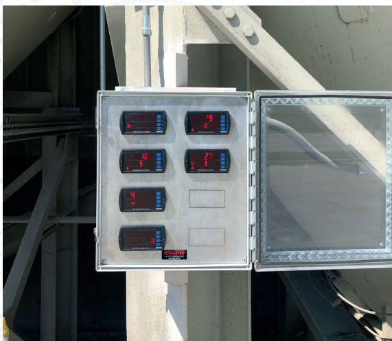
Digital panel meters provide a local display of silo levels to plant personnel.
