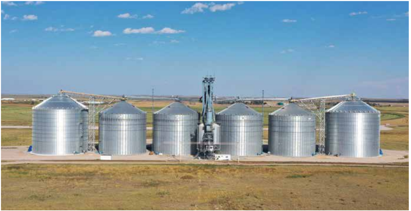
New 675,000-bushel Sukup tanks and yellow AGI Tramco 25,000-bph fill conveyors at far right and far left of the CHS facility at Yuma, CO. Aerial drone photo courtesy of CHS.
