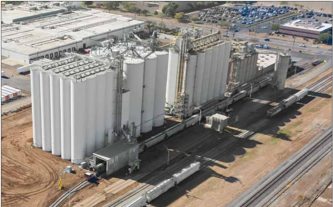
Aerial view of the Bay State Milling Company flour mill in Tolleson, AZ, with new 1-million-bushel elevator annex at far left. Photos courtesy of McCormick Construction Co.
