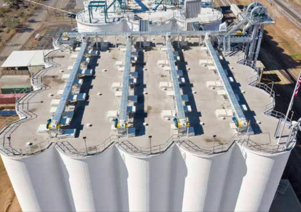
Aerial view of the annex rooftop with 10,000-bph AGI Tramco drag conveyors depositing wheat into 40 upright and interstice bins.
