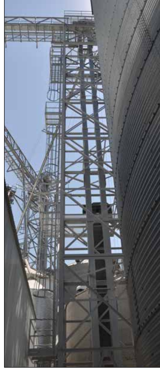
New Schlager 7,500-bph receiving leg allows ingredient receiving and grain drying to be done simultaneously.
