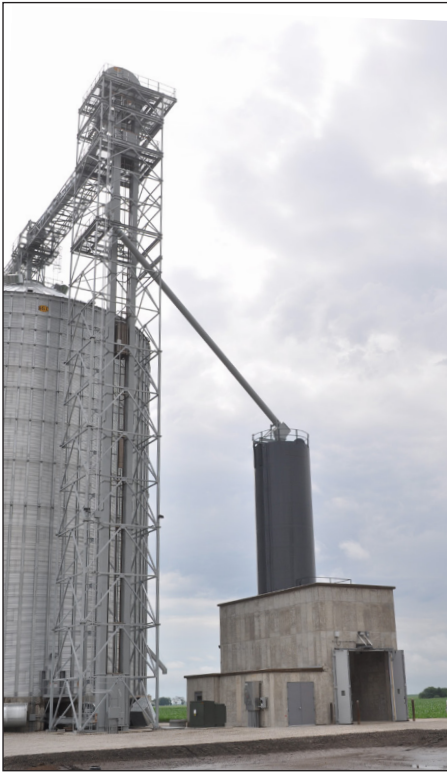
Grain handling equipment includes a 20,000-bph GSI receiving leg at left, with a 1,200-bushel receiving pit in a concrete enclosure and 5,000-bushel Meridian truck-loading surge tank at right.
